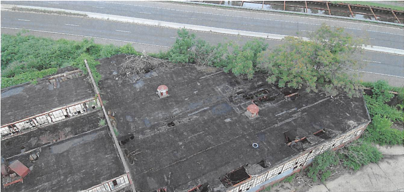
Existing vacant building to be demolished setback to Route 1.
