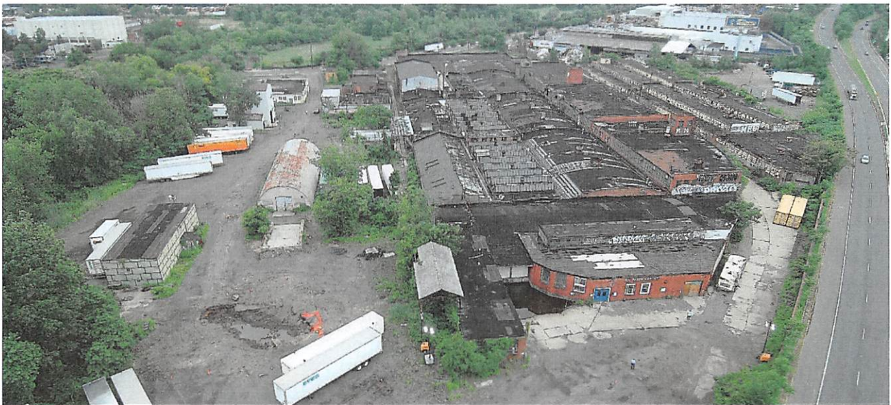
Existing vacant buildings and site improvements to be demolished.
